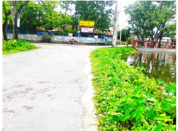
Drain -03, Kumarkhali Pourashava
