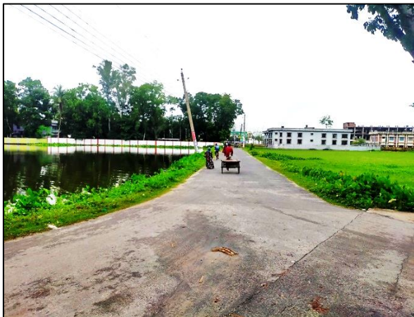
Drain -03, Kumarkhali Pourashava
