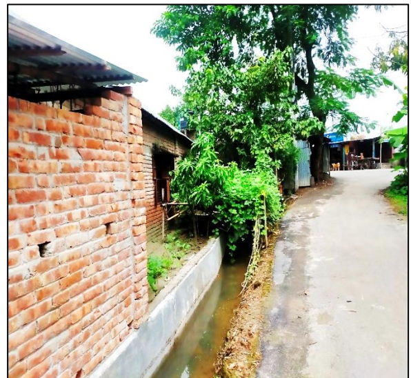
Drain -16, Kumarkhali Pourashava
